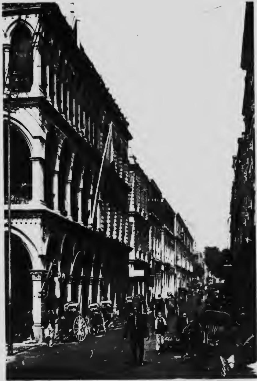
Queen's Road Central, Hong Kong, South China, showing side walks under second stories of buildings so as to afford protection from the sun.
