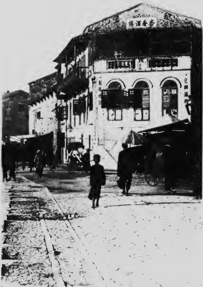
Macao, the Inner Praya. Curious house with bamboo roof garden, oyster-shell windows, brick, tile, and stucco work; architecture showing Portuguese influence of the past five centuries.
