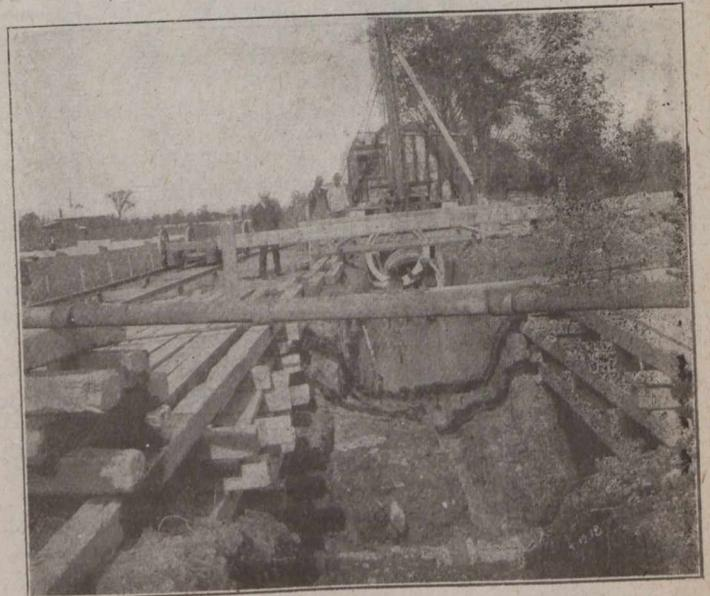
FIG. 5—LAYING 48-IN. CONCRETE PIPE—NOTE CONVEYOR ON TRACK AT LEFT
