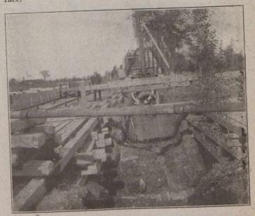
FIG. 5-LAYING 48-IN. CONCRETE PIPE-NOTE CONVEYOR ON TRACK AT LEFT
