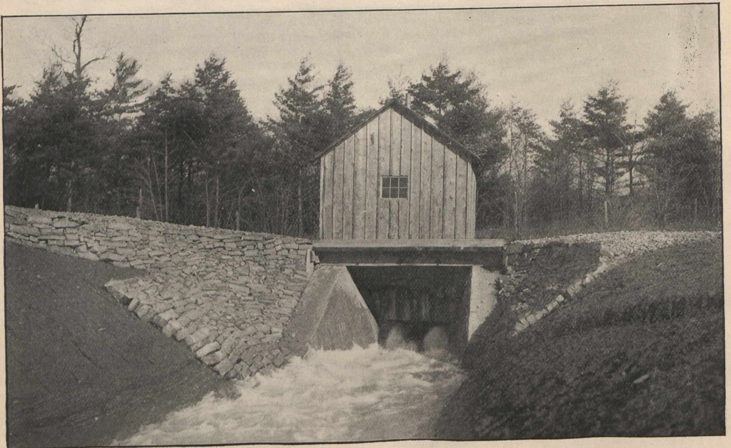
Measuring Weir, City Canal—3,600 cu. ft. per minute.
