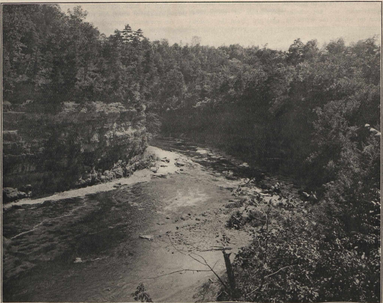
Gorge in Esopus Creek, two miles below site of Olive Bridge Dam. Note shelling character of rock.
