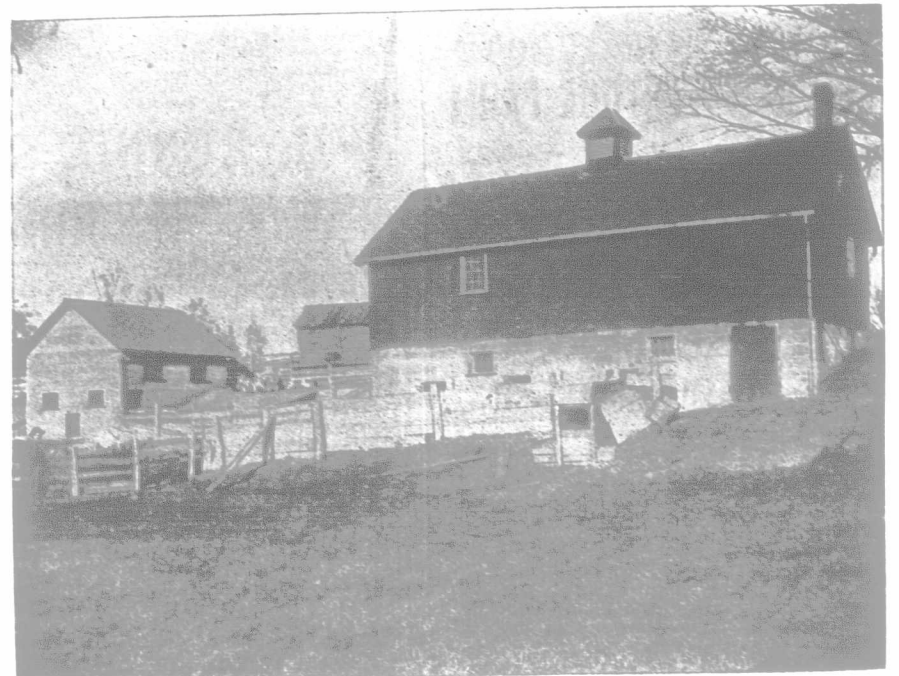
PIGGERY.—Basement walls, floors and troughs built with Thorold Cement, 20 x 40 x 8 feet, one foot thick.
