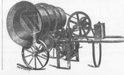
These machines are made to mix either continuously or in batches, and can be operated either by Hand Steam or Gasoline Power.
