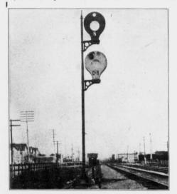
Fig. 22-Disc block signal.
