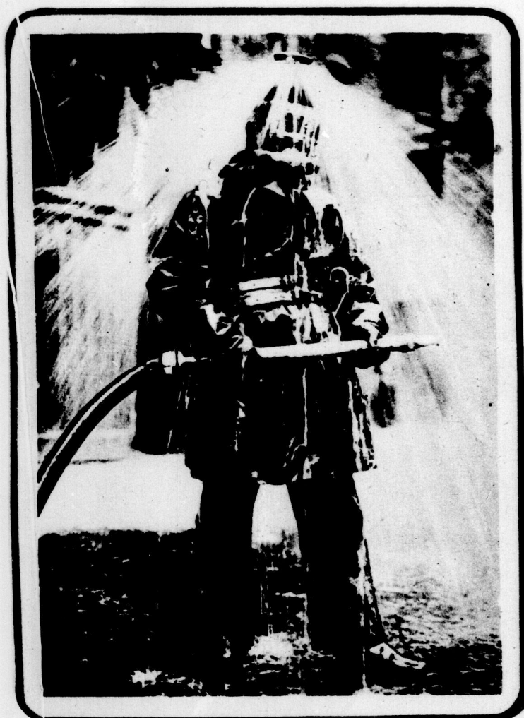
Water-spouting helmet designed to prevent firemen being burned —A European idea
