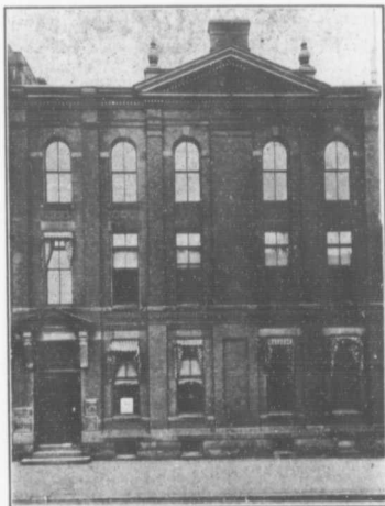
SAINT JOHN BOARD OF TRADE BUILDING, 162 PRINCE WILLIAM STREET
