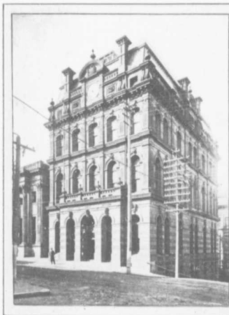
POST OFFICE, PRINCE WILLIAM STREET
