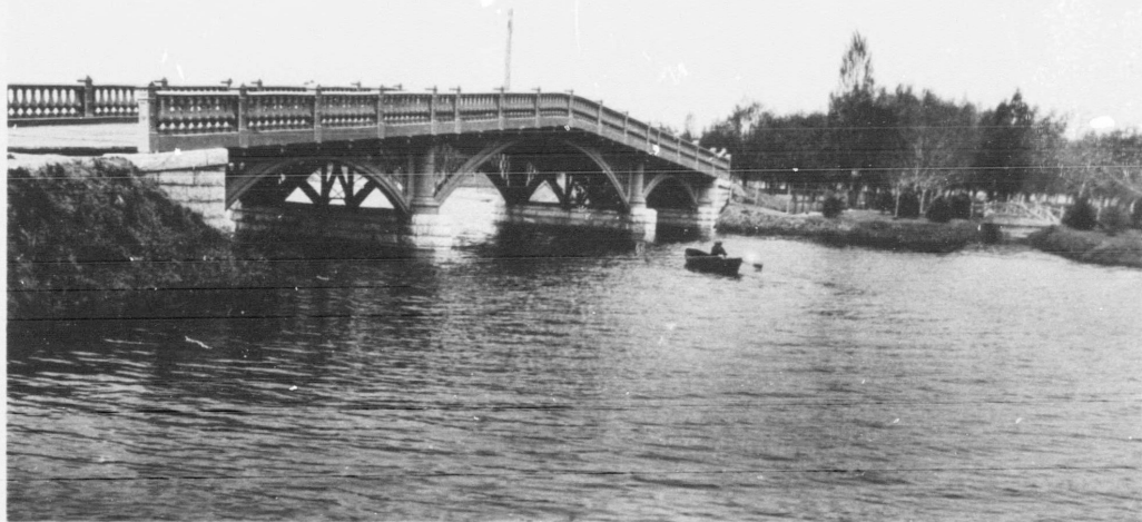
HALLAM BRIDGE—ISLAND PARK.
