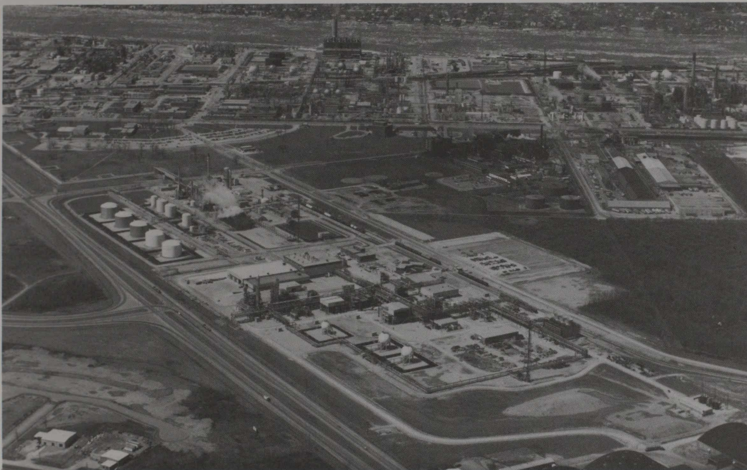
Polysar's headquarters and plant in Sarnia, Ontario. A drawing of this plant graced the back of the Canadian $10 bill until 1986.
