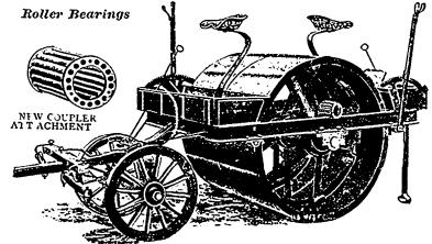
With Roller Bearings and New Patent Coupler Attachment, either 21/3, 31/3, 41/4 or 51/2 tons. All one size frame, drum, and, width of tread and can be extra weighed 2 tons each. Address for Catalogue
