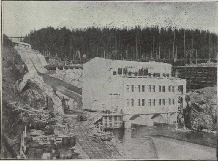
Fig. 3.—The Power House, Showing Two Penstocks and Tailrace Weir.
