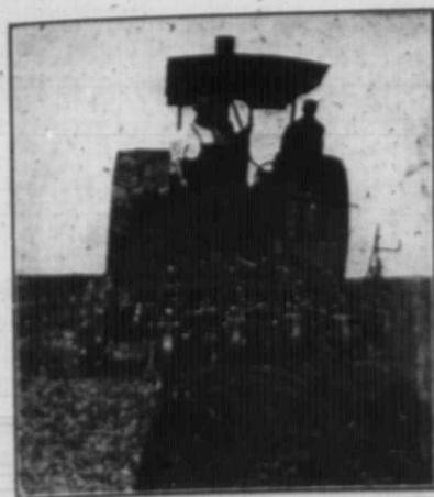
Marshall, Sons & Co. Saskatoon, 2 cylinder, 35 h.p. all tractor pulling two 14-inch plows.
