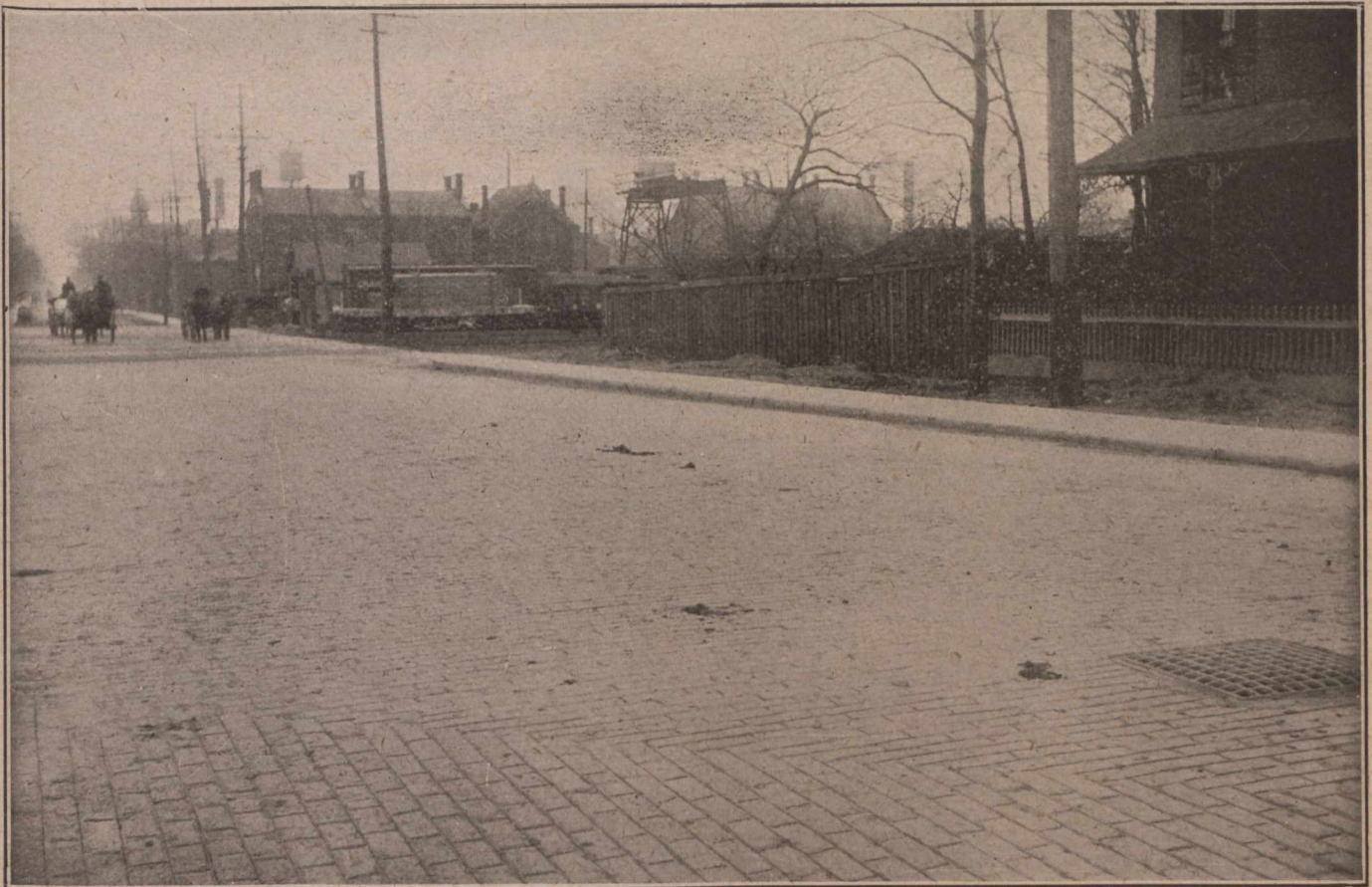
BRICK PAVEMENT ON CANNON STREET, AT ELGIN STREET, HAMILTON
