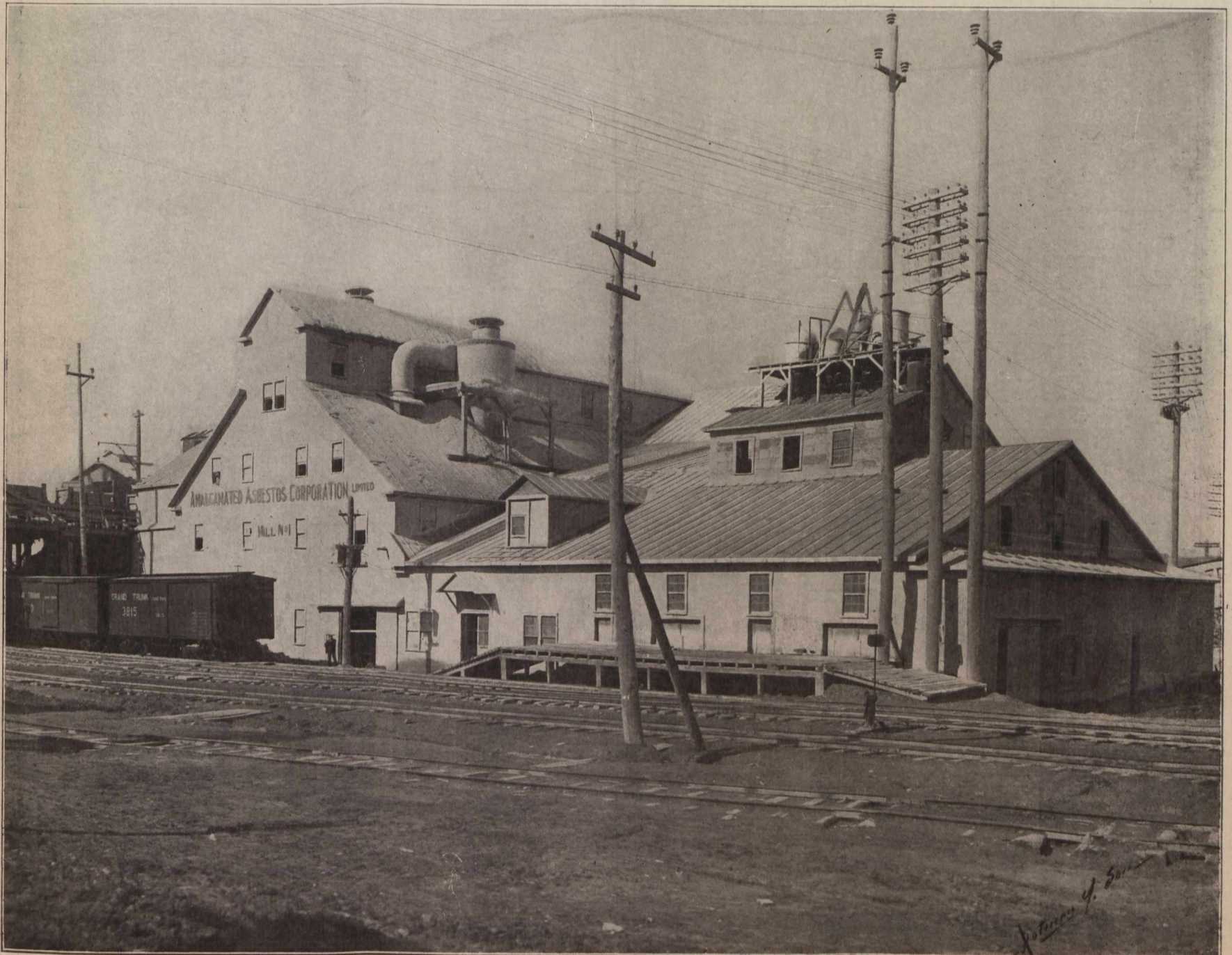
Asbestos Mill of the Asbestos Corporation of Canada, Limited, Thetford Mines, Quebec.
