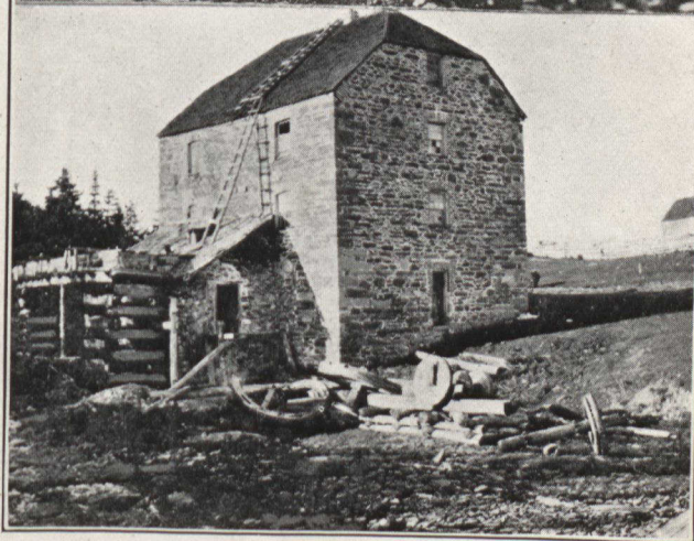
1. PORT DANIEL TUNNEL.—Showing train. 2. DAY'S MILL.—Bonaventure.
