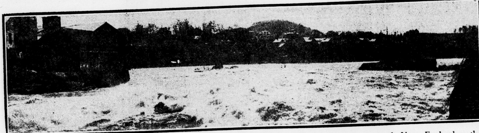
Houses undermined, highways flooded and bridges threatened are the conditions in various parts of New England as the Connecticut and Merrimac rivers race through four states in the flood stage brought on by melting snows
