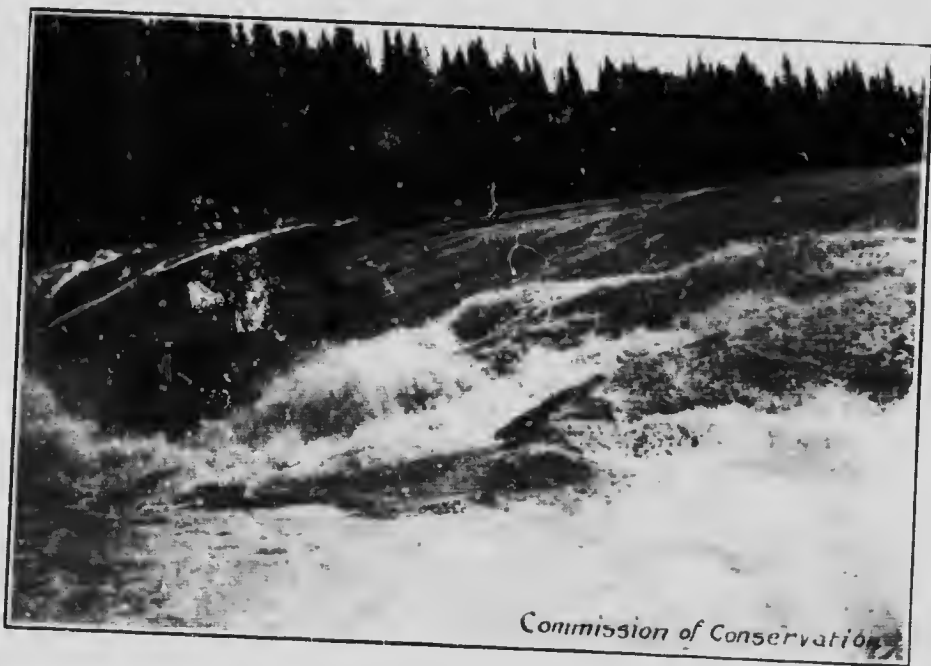
NELSON RIVER—WHITEMUD FALL (WEST CHANNEL)
