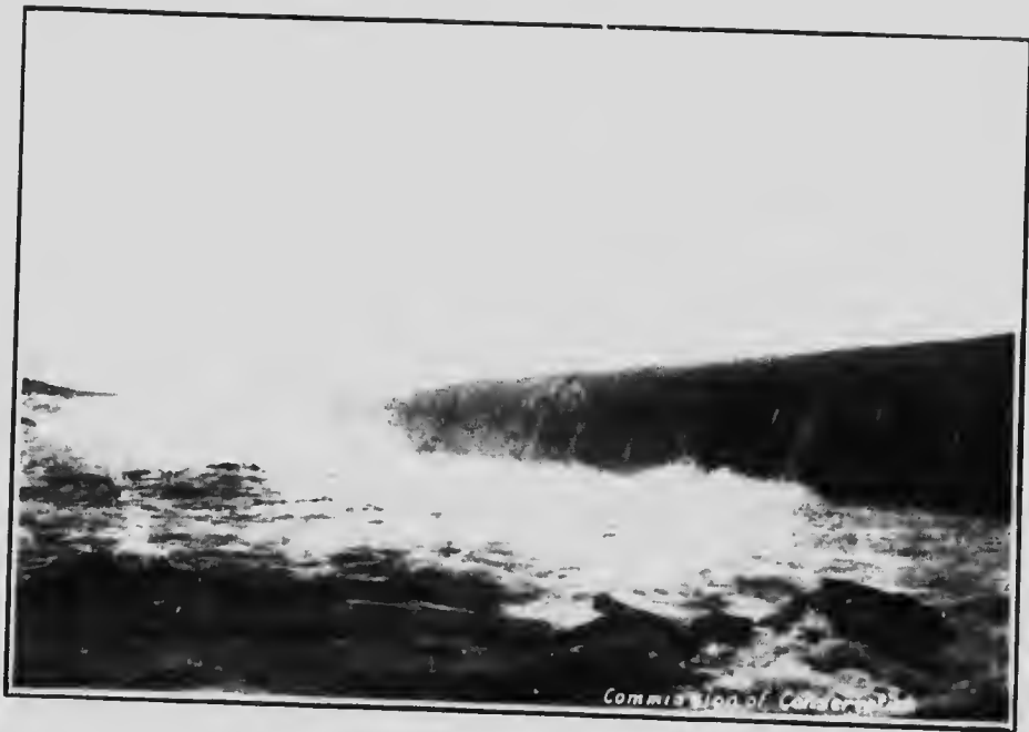
WINNIPEG RIVER - SPILLWAY OF POINTE DE BOIS PLANT
