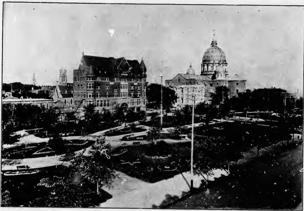
THE NEW ST. PETER'S CATHEDRAL, MONTREAL, has been building so long that it is scarcely entitled to the adjective, although it is not yet completed. It is twenty-five years since the structure was commenced, and the work has gone on uninterruptedly, although slowly, ever since. The plan of the architecture is fashioned after the historic St. Peter's at Rome, with an immense dome in the centre of smaller surrounding domes. It is a massive structure of grey stone, and when completed will be the largest church on the continent. To build it has been a colossal undertaking, but the end is now near. The frescoers have been at work the past year and the dedication will take place within a few months. The other large building shown in the picture is the home of the Young Men's Christian Association. It is almost new, having been completed only two years ago. Its cost was $185,000, and it is, with the exception of the building at Brooklyn and the new one just finished in Chicago, the largest Y.M.C.A. building on the continent.
