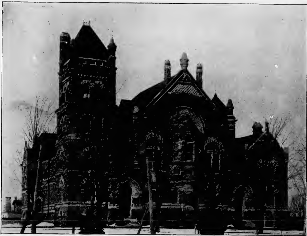
OXFORD COUNTY COURT HOUSE. WOODSTOCK, ONT. —The new county buildings of Oxford, shown in the engraving, are said to be the finest in the Province of Ontario. They suitably represent the wealth and substantial prosperity of the richest cheese county in cheese-producing Canada. They also appropriately testify to the progressiveness of the town of Woodstock, one of the most thriving and up-to-date towns in Canada, and one whose growth during the past six or seven years, has been equalled by only one or two of its competitors.
