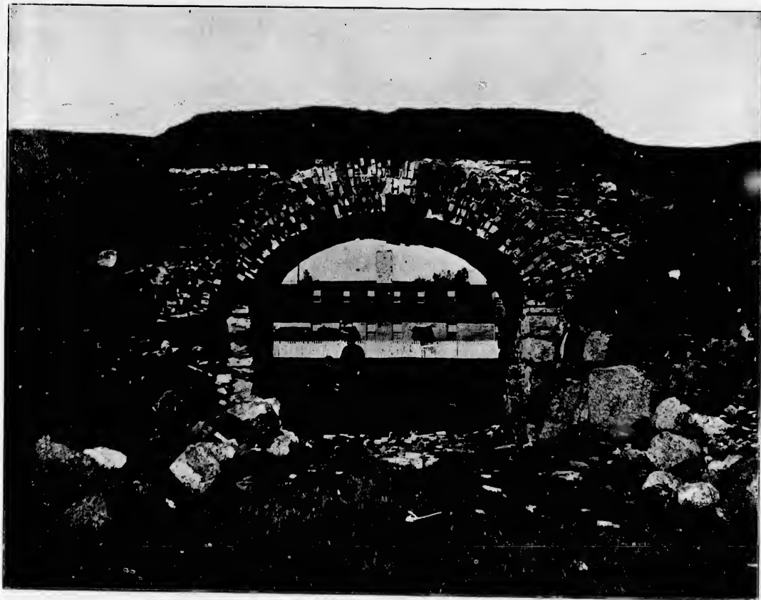
SALLYPORT, FRENCH FORT, ANNAPOLIS. —The old fort occupies a peninsular piece of land where the basin of Annapolis suddenly contracts like the neck of a bottle. The trenches and earthworks are covered with grass, and the trees in the corners of the excavations show signs of decrepitude. A part of the loose stone wall with which the parapet on one side was faced still remains, and the arched sallyport is in a moderately good state of preservation. The wooden building standing in the centre of the quadrangle was used as a barracks in the days of the fort's vigor. There is a small stone building in a corner of the earthworks. It was the magazine of the French and is said to have been built in the year 1642. Near by is the old grave yard in which the soldiers who used to garrison the fort lie buried.
