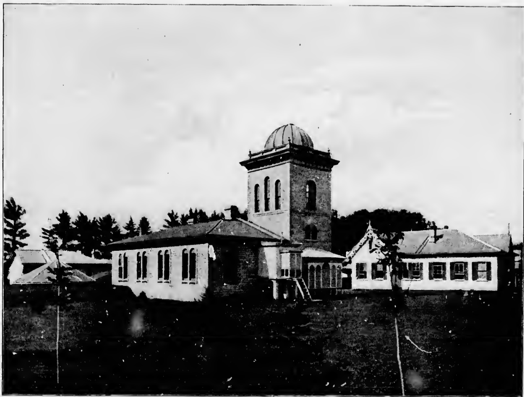
TORONTO MAGNETIC OBSERVATORY. —The weather factory, as the building in the engraving is facetiously called, excites a great deal of interest throughout the Province of Ontario, and even the other provinces of the Dominion. From this low glass-domed building go out the daily weather "probs" by which, to a greater or less degree, the affairs of the Dominion are governed. But in addition to this popular part of the observatory it has functions of a scientific and national character with which, however, the ordinary individual has little interest. The building, with the others connected with it, is situated close to the Provincial University in Toronto.
