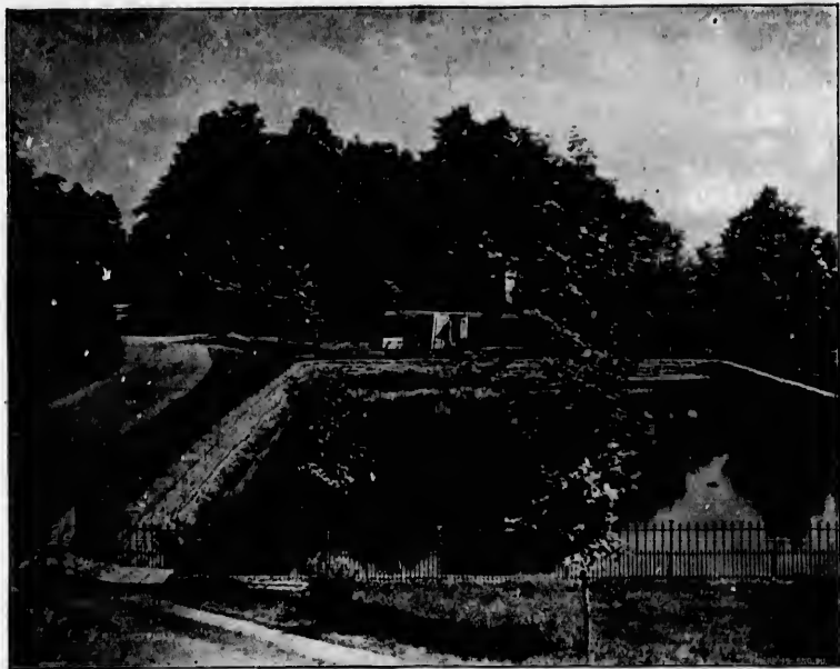
HIGH LEVEL RESERVOIR, MONTREAL. —In connection with the water supply there are two points of interest for visitors to the city. One is the general city reservoir, which is hewn out of the solid rock far up the mountain side, its capacity being 36,500,000 gallons. It is supplied by an aqueduct which leads the water of the St. Lawrence from above the Laclaire Rapids to a point on the western limit of the city, where it is pumped up the mountain to the reservoir. The other is the High Level Reservoir, picturesquely situated in Mount Royal Park, higher than the general city reservoir and just adjoining the splendid residence and grounds of the late Sir Hugh Allan, founder of the Allan steamship line. To reach the summit of the mountain from this reservoir there is a graduated flight of steps up the face of the cliff, the reward for the climb being a beautiful variety of landscape views and a view of the city and river below.
