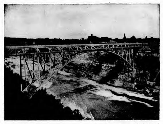
THE LOWER STEEL ARCH BRIDGE.—What is known as the Gorge is crossed at its narrowed point by an arch bridge built in 1897 by the Grand Trunk Railway. The arch is of 550 feet span, and supports two roadways, the topmost for trains, and the lower for wagons. A fine view of the Rapids may be had from this bridge.
