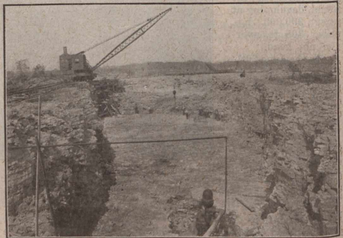
CRANE MOVING ROCK IN SKIPS FROM CANAL SECTION AT ENTRANCE TO FOREBAY
