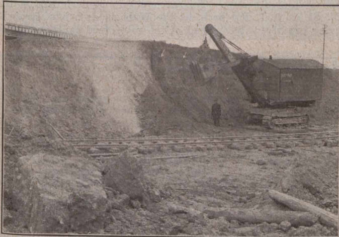
7/8-YD. SHOVEL AT THE G.T.R. AND M.C.R. DIVERSION
