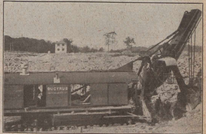
4 1/2-YD. SHOVEL IN ROCK AT THE FOREBAY
