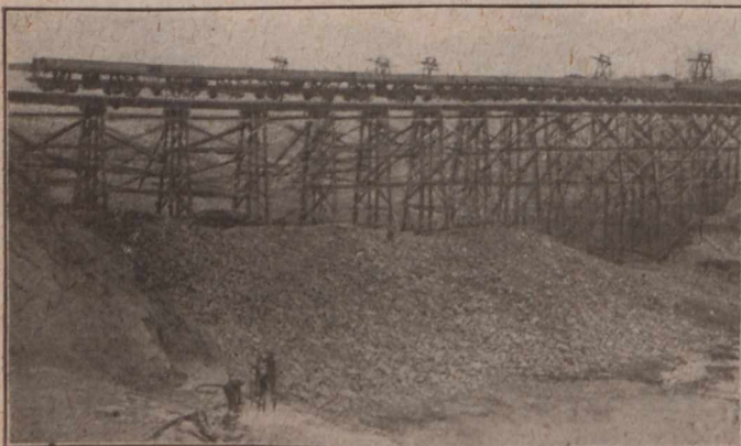
DUMPING ROCK FROM TRESTLE FOR FILL AT THE WHIRLPOOL GULLY
