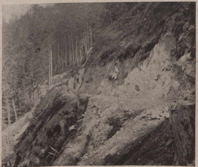
Fig. 3.—View Showing Rough Nature of Ground Over which Pipe Line was Constructed.
