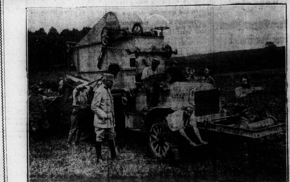
WONDERFUL TRENCH DIGGER This photograph gives a good idea of the marvellous trench-digger being used by the French to dig their lines in the recaptured districts. This machine not only digs a uniform trench many miles long in quick order but also erects a satisfactory ramp part as it goes along.
