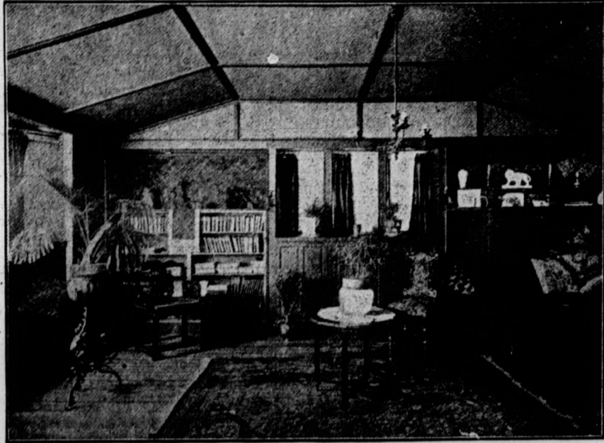
CEILING OF ARTIST'S DEN FINISHED WITH WALL BOARD
