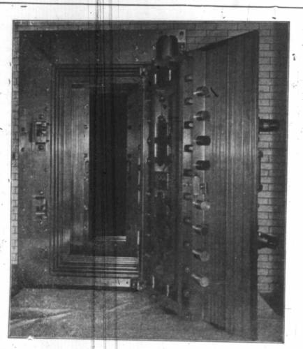
Vault doors in Bank of Montreal and Royal Trust Company, Morgeal Three times larger and heavier than any other in Canada. Doors and Vestibules weigh 60 tons. Total weight of lining and doors 260 tons. Accepted to be the finest piece of vault work in construction and workmanship in the Dominion. — Built by the old established firm of
