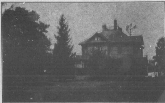
A County Home that is Attractive Without and Convenient Within
