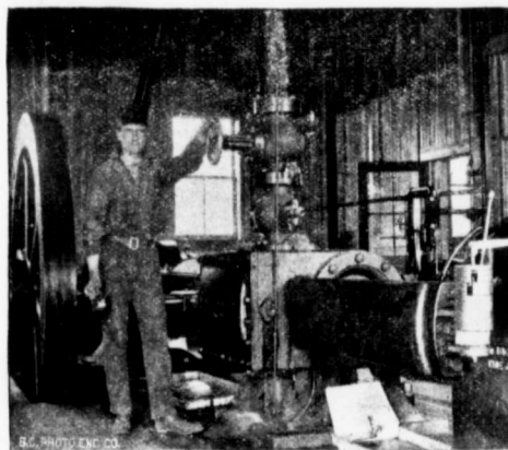
INGERSOLL-SERGEANT AIR COMPRESSOR AT SUNSET MINE.
