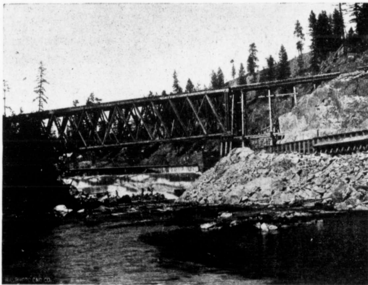
DAM AND HEAD OF FLUME, GRANBY SMELTER.
