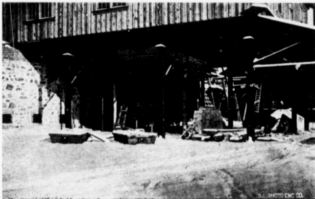
FURNACE IN COURSE OF CONSTRUCTION, B. C. CO'S SMELTER.
