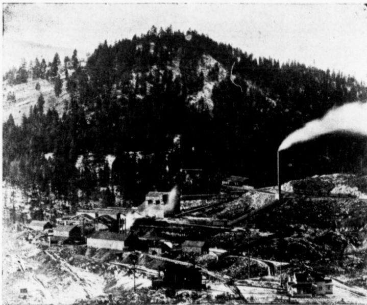
B. C. COPPER CO'S SMELTER, NEAR GREENWOOD, B. C.
