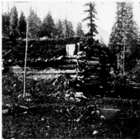
FIRST PROSPECTOR'S CABIN ON BOUNDARY CREEK. (Built in '86).
