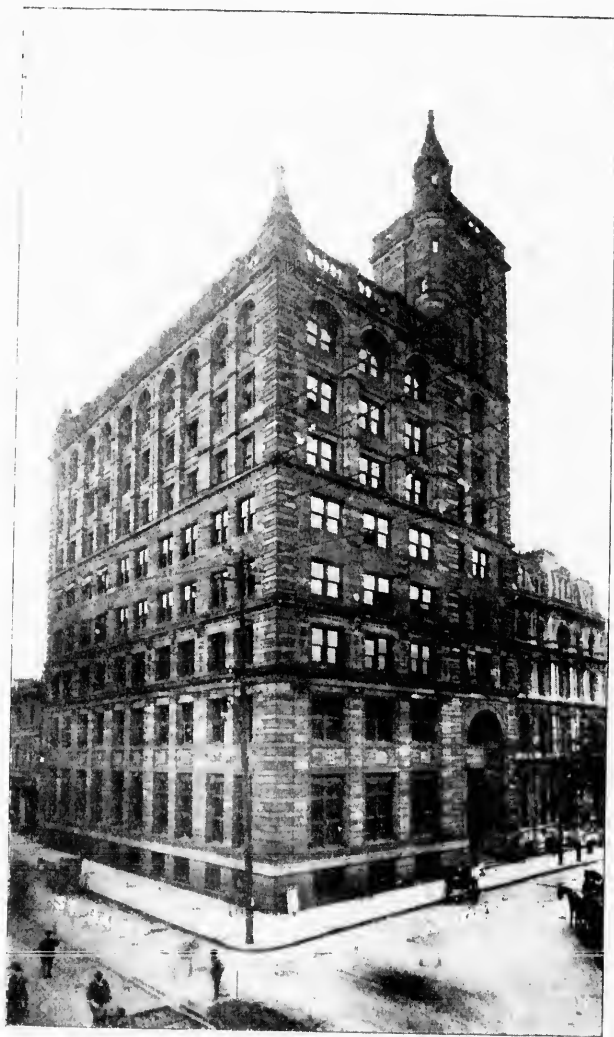
MONTRÉAL OFFICES: NEW YORK LIFE BUILDING.
