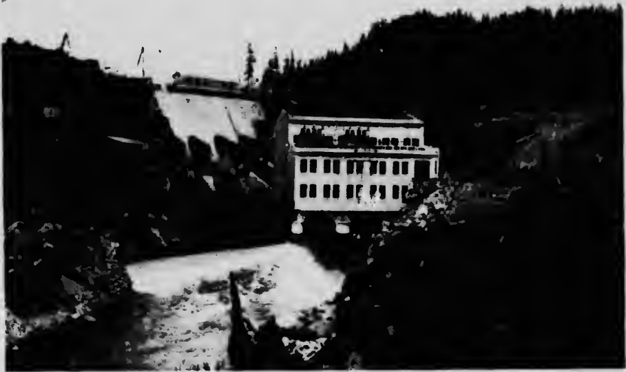
Stave Lake Development. Power House, Stave Lake.
