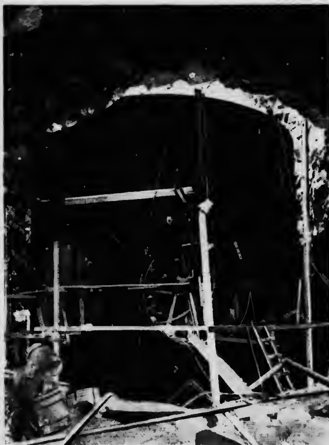
Coquitlam-Buntzen Development. Surge tank, showing openings for pipe line connections.
