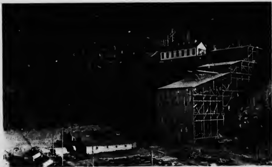
Britannia Mining and Smelting Company Limited. New Reduction Mill, with Beach Power House in rear and Beach Compressor House in foreground. The Aerial Tramway is seen on the side of the mountain.
