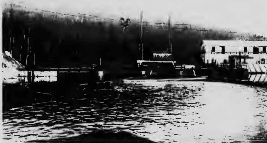
Stave Lake Development. Looking downstream above dam.
