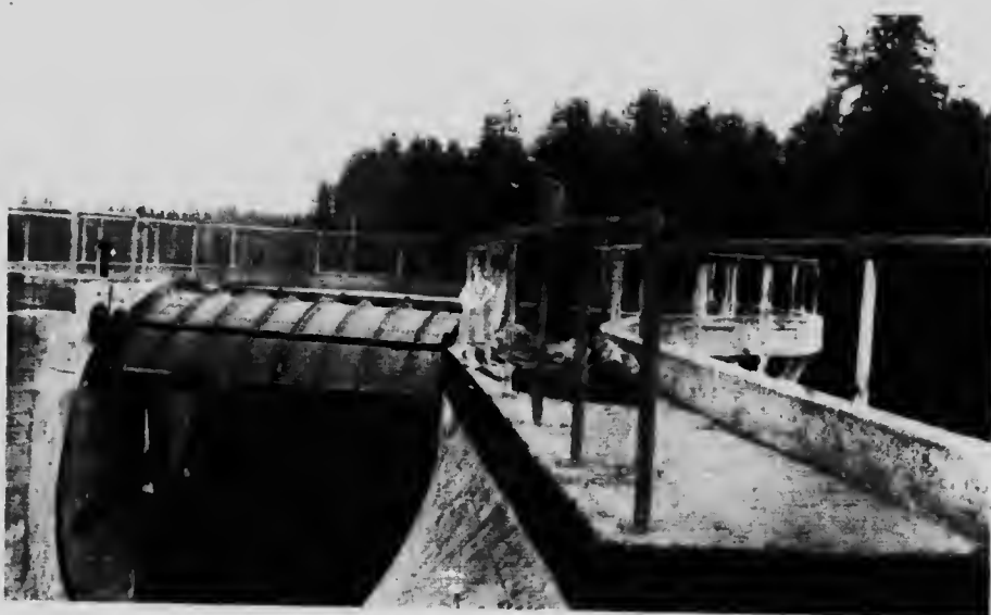
Canadian Collieries (Dunsmuir) Ltd. Forebay, showing Screens and Tainter Gate in open position.
