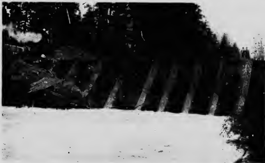
Canadian Collieries (Dunsmuir) Ltd. View showing downstream face of Storage Dam.
