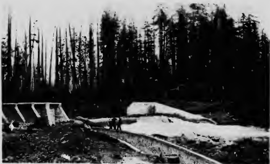
Canadian Collieries (Dunsmuir) Ltd. Diversion Dam.
