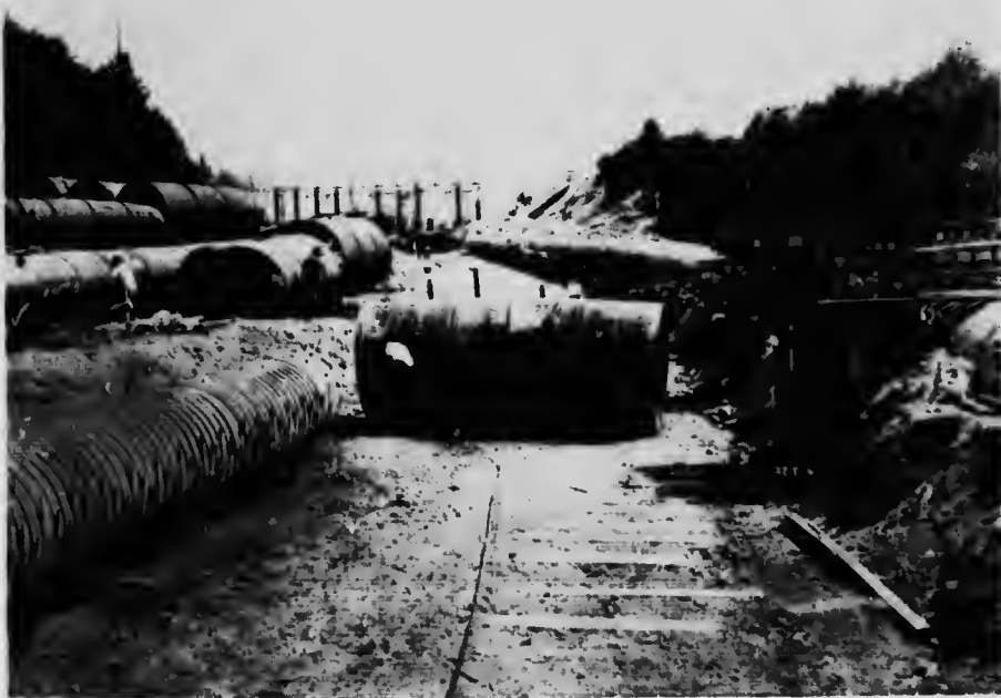
Coquitlam-Buntzen Development. Replacing wood stave pipe lines with rivetted steel pipes.
