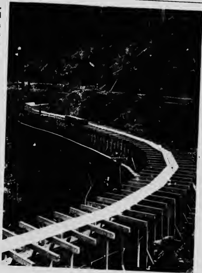
Vancouver Island Power Company Limited Flume and Railroad above Forebay.
