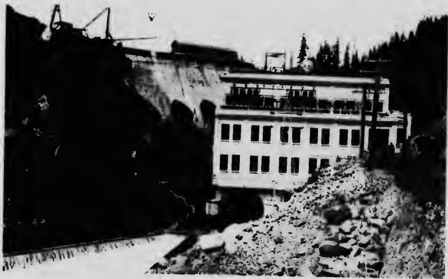
Stave Lake Development. Stave Falls Power House.
