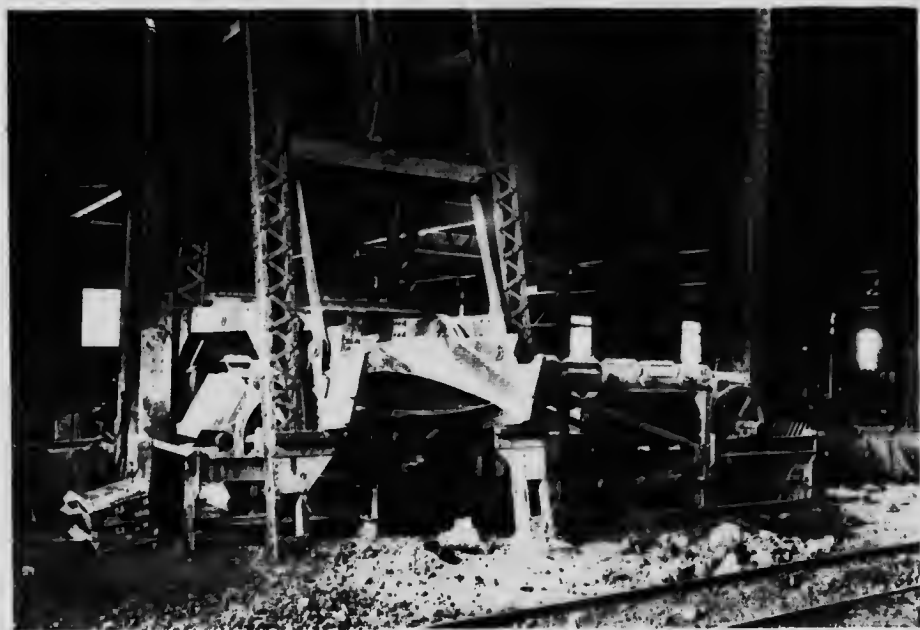
Granby Consolidated Mining, Smelting and Power Company Limited. Casting Machine.
