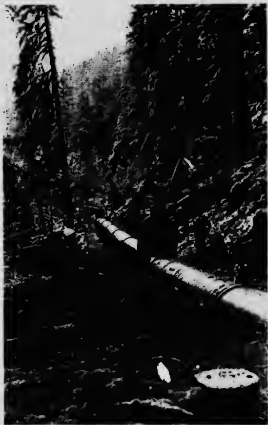
City of Prince Rupert-Woodworth Lake, near Prince Rupert. 45 inch Pipe Line with 45 inch Valve in position.
