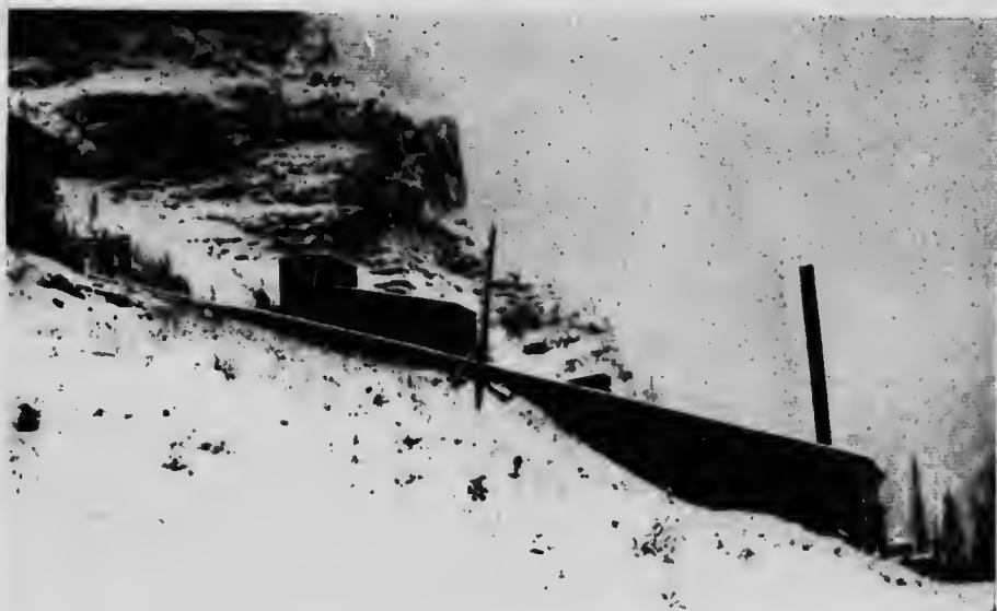
Cathedral Creek Development. Concentration Plant and Power House, Mount Steven Mine.
