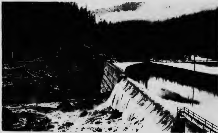
Vancouver Island Power Company Limited. Jordan River Dam with water passing over spillway.
