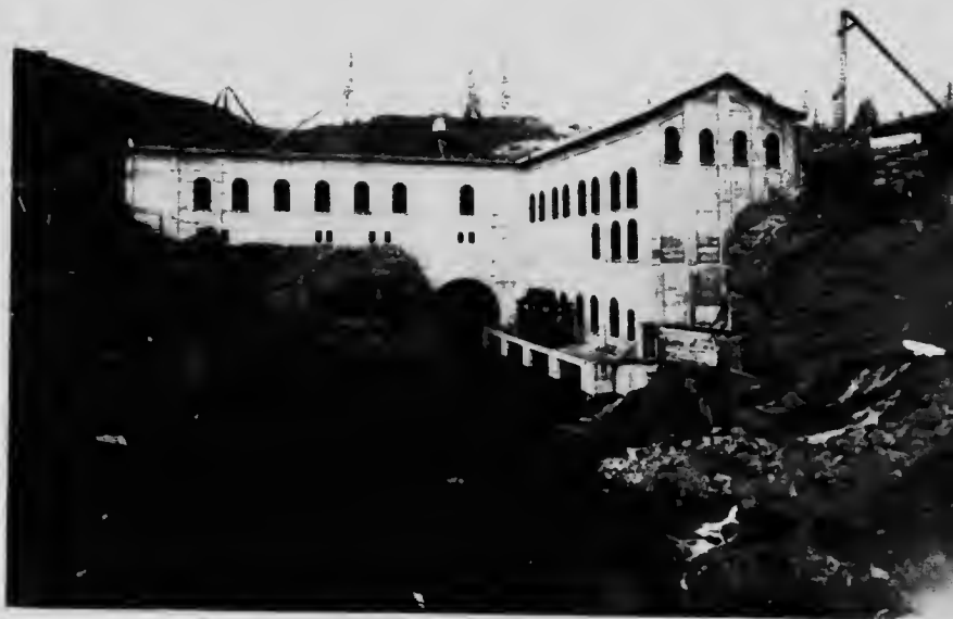
Kootenay River Development, Bonnington Falls. Front View, No. 2 Power House, Upper Bonnington Falls.
