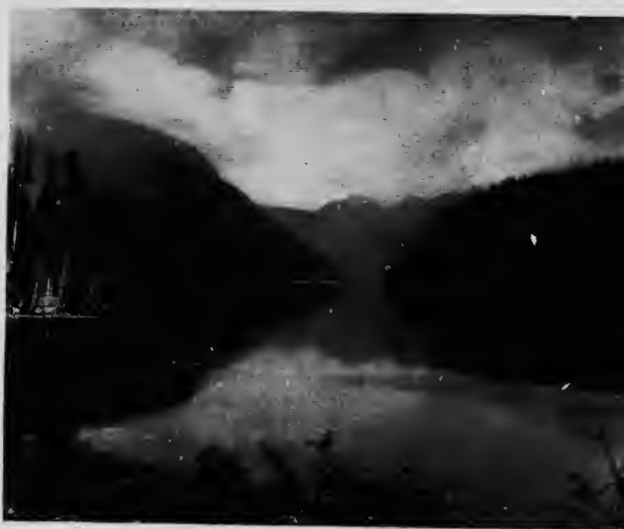
Coquitlam-Buntzen Development. Coquitlam Dam.
