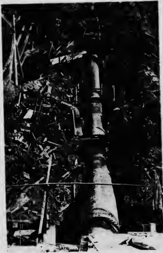
Vancouver Island Power Company Limited. No. 3 Pipe Line as seen from Power House.
