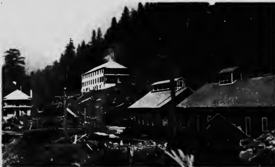
Britannia Mining and Smelting Company Limited. Tunnel Camp. Britannia Mine. Tunnel Power House (in centre) Dormitory and Machine Shop.
