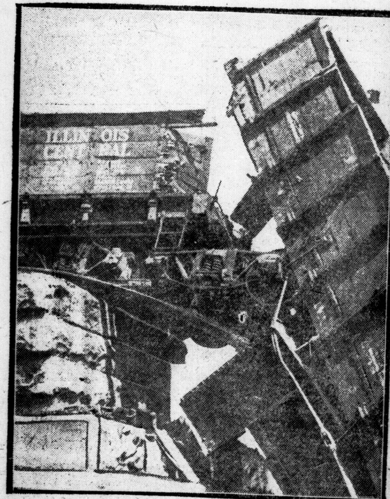
A steel trestle unexpectedly collapsed in Indianapolis with the result that eight freight cars dropped thirty feet into the creek beneath.
