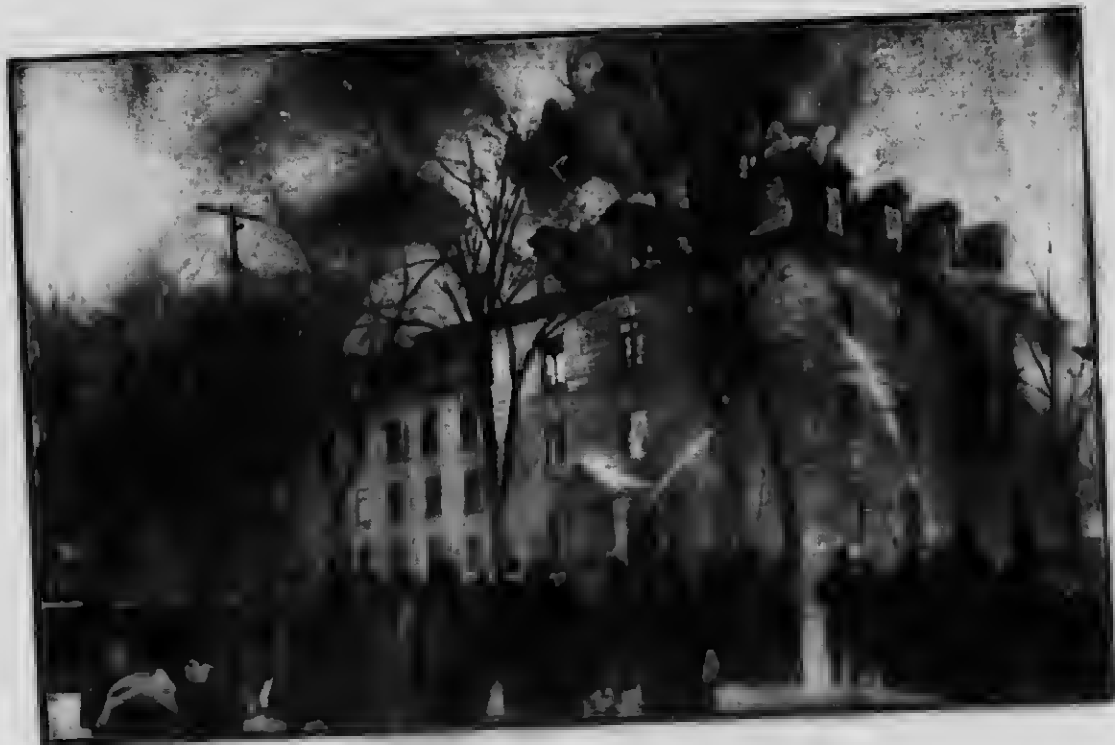
Where the fire started, University of Ot'awa.
