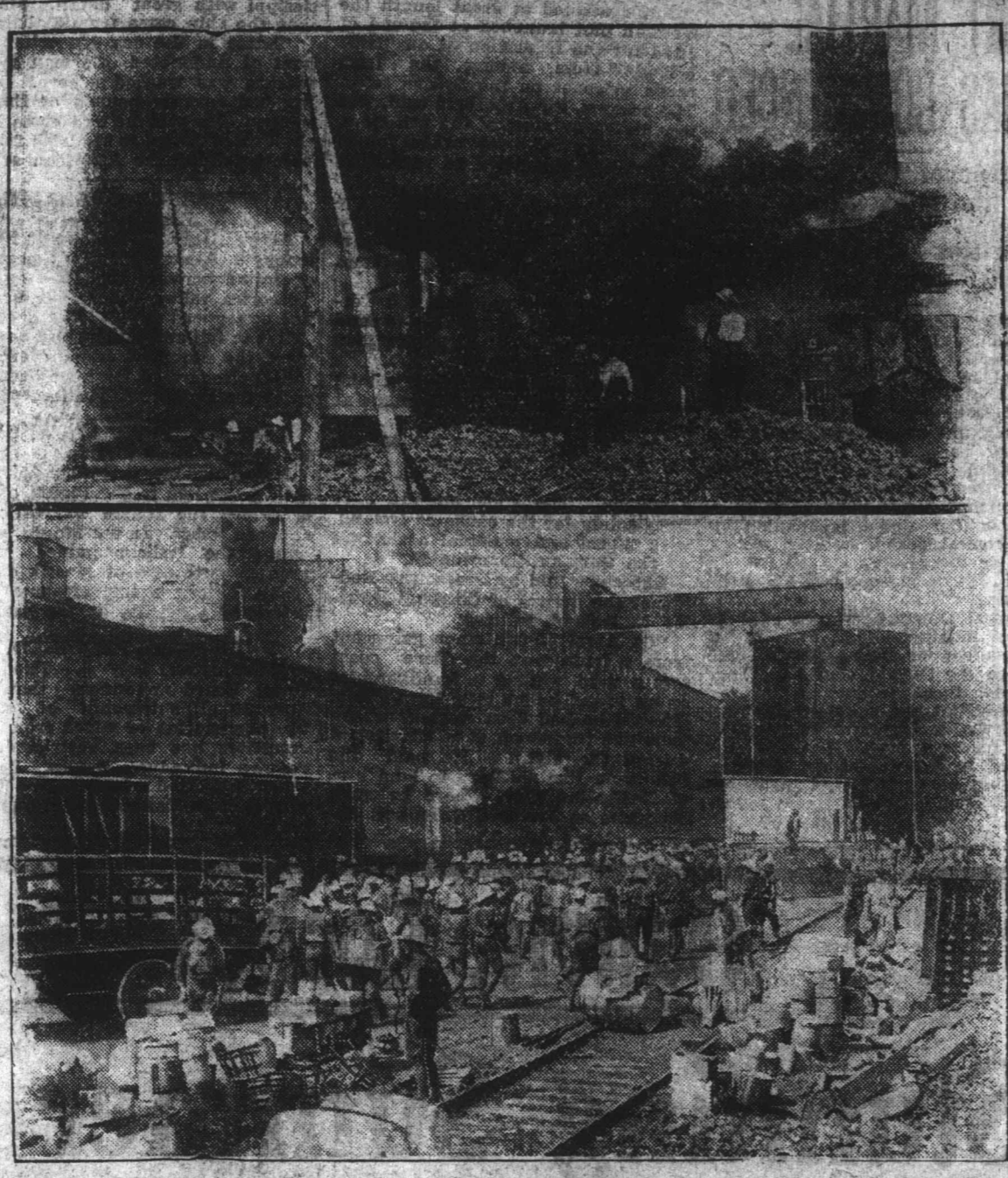
AVIATION CADETS AID FIRE-FIGHTERS IN SAVING CONTENTS OF PORT CREDIT STARCH WORKS. The older section of the Port Credit Starch Works, known as plant No. 2, was damaged to some extent of over $100,000 Thursday afternoon by fire. The contents of damaged by water and smoke. Cadets from Long Branch rendered in tents of the building. The photograph was on the spot during the interesting pictures.
