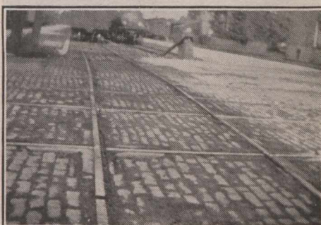
Trussed Rail Joint, London Street Railway.
