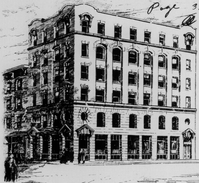
Home of the Leeming Miles Co., Limited, Corner Notre Dame and St. Lambert Sts., Montreal.
