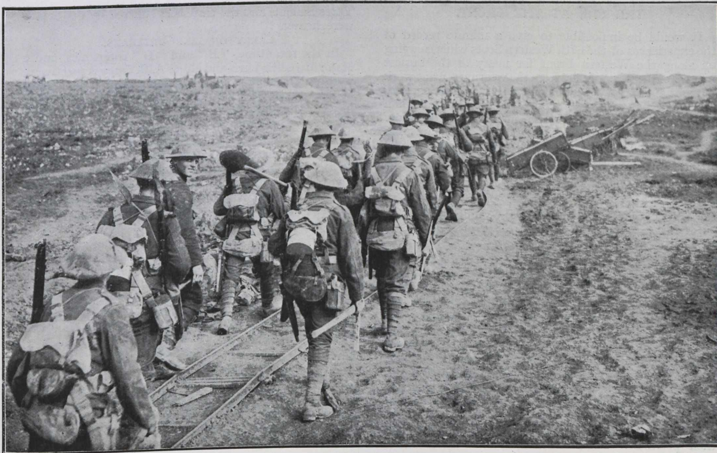
Work for the Pioneers: Going into the Somme with picks and shovels during the memorable days of 1916.
