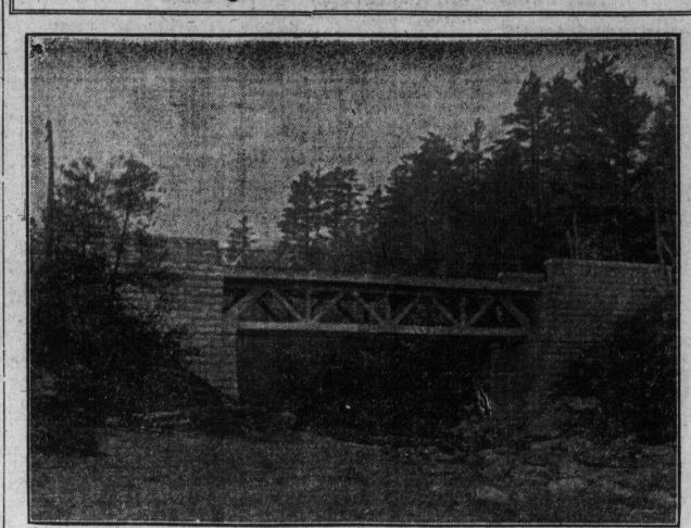
The above cut shows a bridge on Kingston road over Highland Creek, which had to be repaired strengthened this last summer. County Engineer Frank Barber was entrusted with the work, and instead of discarding the old steel superstructure, he surrounded each member of the bridge with concrete, which now has the durability of a new reinforced concrete bridge. The span of this bridge is 60 feet and the floor is 32 feet
