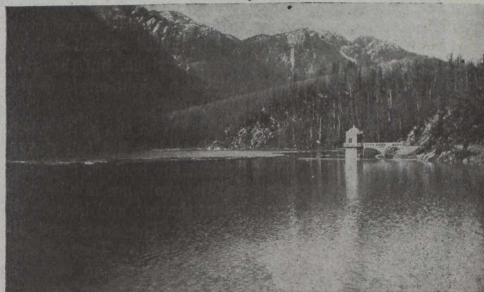
Fig. 6.—Water Tower with Lake Level Raised.
