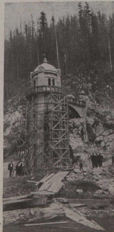
Fig. 7.—Water Tower, Front View.
