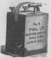
The strongest and most powerful machine ever made for Electric Blasting. No. 3 fires 30 holes; No. 4 fires 50 holes; No. 5 fires 100 holes. They are especially adapted for submarine blasting, large railroad quarrying, and mining works.
