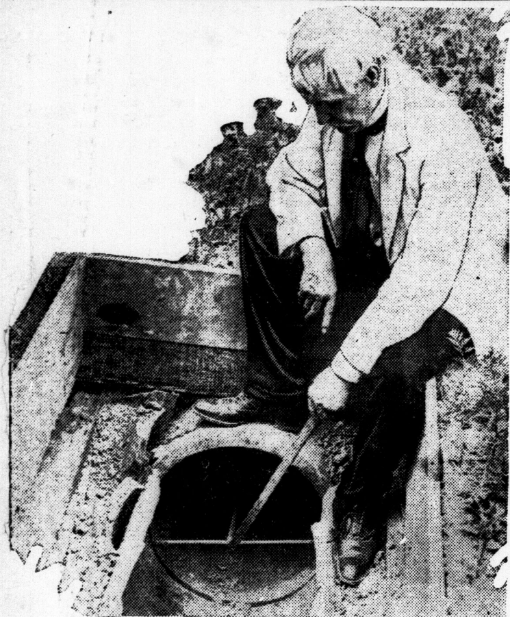
Dr. James Rogers, Maryland experimenter, and his underground antenna, by which he transmitted a message to Toulon, France. He is the originator of the theory that long distance radio waves travel through the earth and sea rather than through the air
