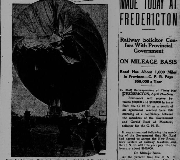
Here is shown the first photo of the giant Dirigible R-33, which tore loose from her moorings at Fulham, England, by a terrific wind storm and, after twenty-four hours buffeting about over the North Sea, was guided back to her hangar. The picture shows clearly the damage sustained to the big ship's nose when she broke away.
