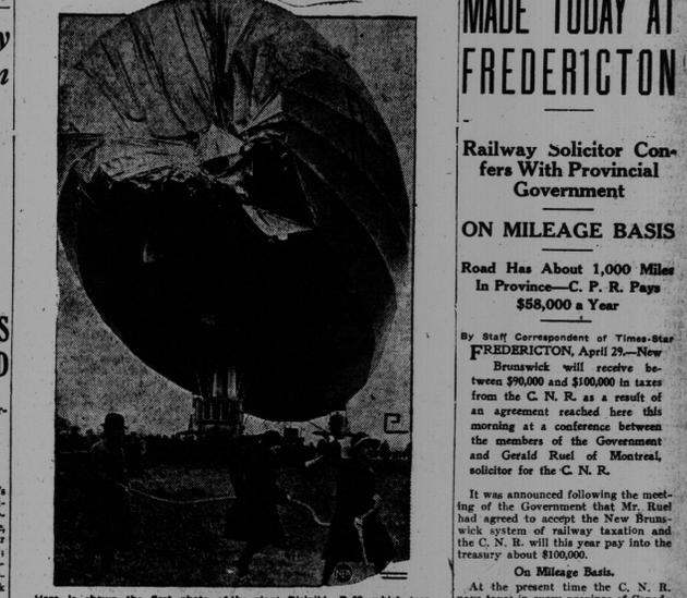
Here is shown the first photo of the giant Dirigible R-33, which tore loose from base moorings at Puffin, England, by a terrific wind storm and, after twenty-four hours buffeting about over the North Sea, was guided back to her hangar. The picture shows clearly the damage sustained to the big ship's nose when she broke away.
