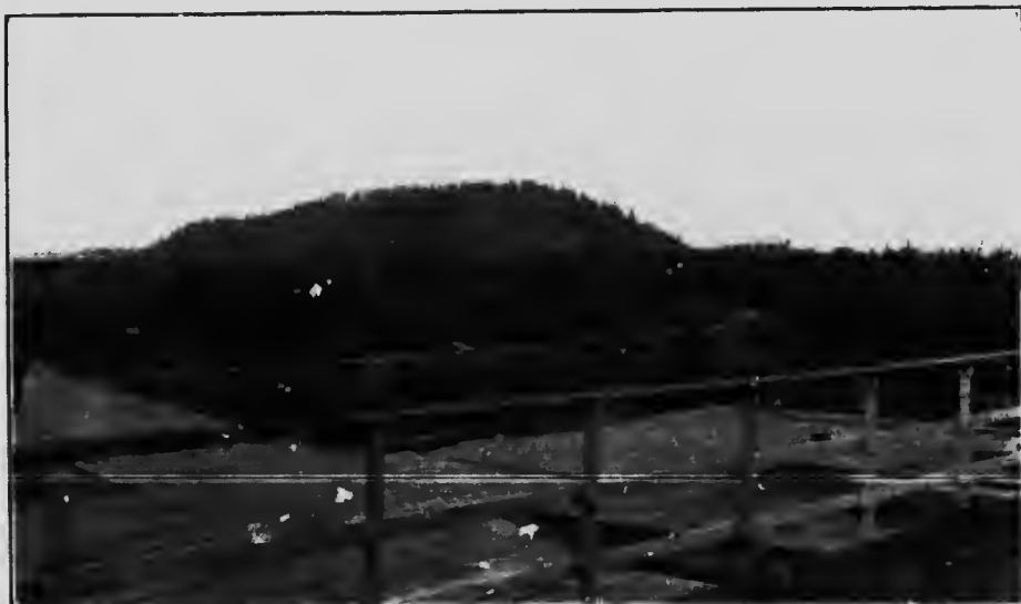
Reclamation-Pitt Meadows Dyke South of Sturgeon Slough.
