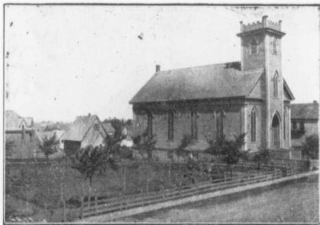
THE SECOND BUILDING Built in 1863.
