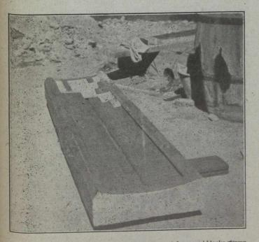
Showing concrete retainer for wood block diffusers. A few wood blocks shown in place. Blocks ½" thick and from 2½" to 4" square.
