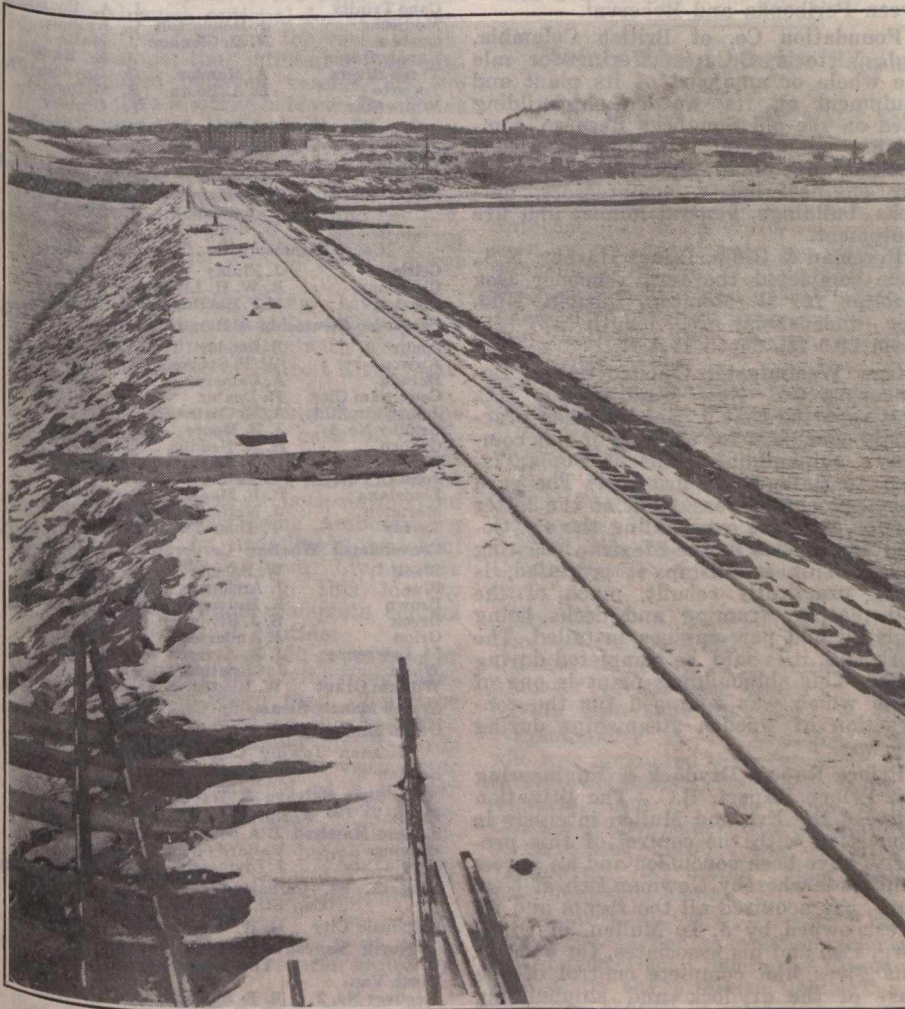
Looking along top of Breakwater at Courtenay Bay, St. John, N.B.
