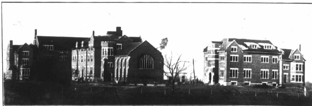
New Dormitory Building for Boys and Married Masters' Residence, Ridley College, St. Catharines, Ont.
