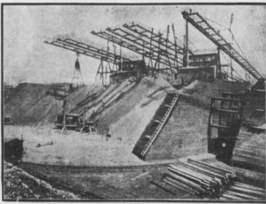
Fig. 153—Unloading ore from Lake Steamers. This ore is brought from the mines and transferred from the boat to the dock by huge steel cranes
