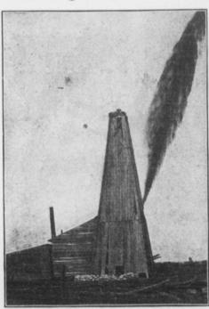
Fig. 105—Torpedoing an Oil Well near Petrolea, Ont. face.
