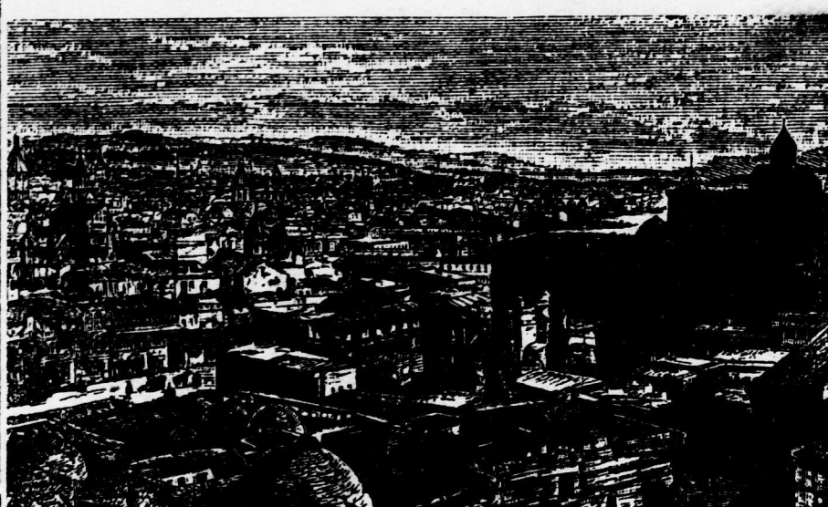
THE CITY OF TIFLIS. TRANS-CAUCASIA. An entire township in the immediate vicinity of the city has been destroyed by an avalanche.
