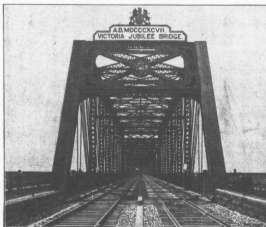
PORTAL OF GRAND TRUNK RAILWAY, VICTORIA JUBILEE BRIDGE OVER ST. LAWRENCE RIVER, MONTREAL.
